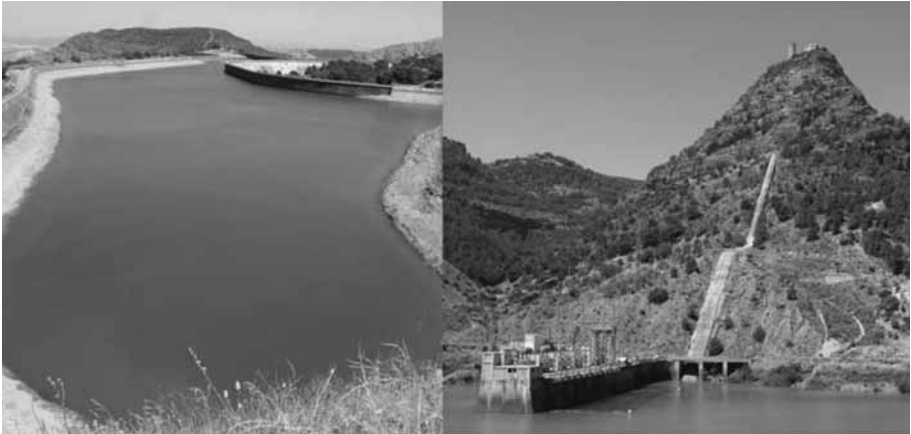
Note: Left: Upper Reservoir; Right: Lower Reservoir, Penstock and Surge Shaft
