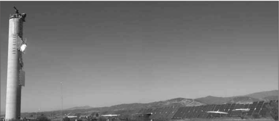
Figure 1.11 Demonstration Solar Thermal Tower Power Plant in Spain
