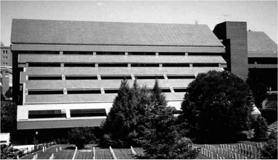
Figure 4.1 Roof-integrated Photovoltaic System [Georgetown University in Washington (USA), Installed in 1984 with 4464 Photovoltaic Modules and 337 kW p Total Power]
