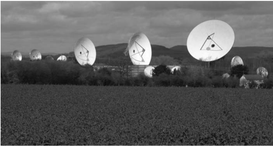
Figure 8.44 Madley communications centre (Copyright Philip Halling)
